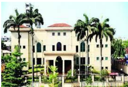
Fig. 1: Muson Centre, Onikan-Lagos Source: https://muson.org
